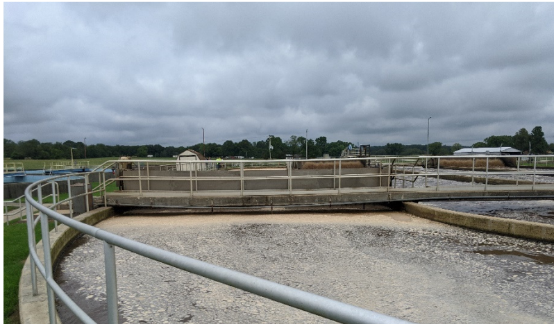
Figure 2-10: Aeration Basin Sagging Bridge
