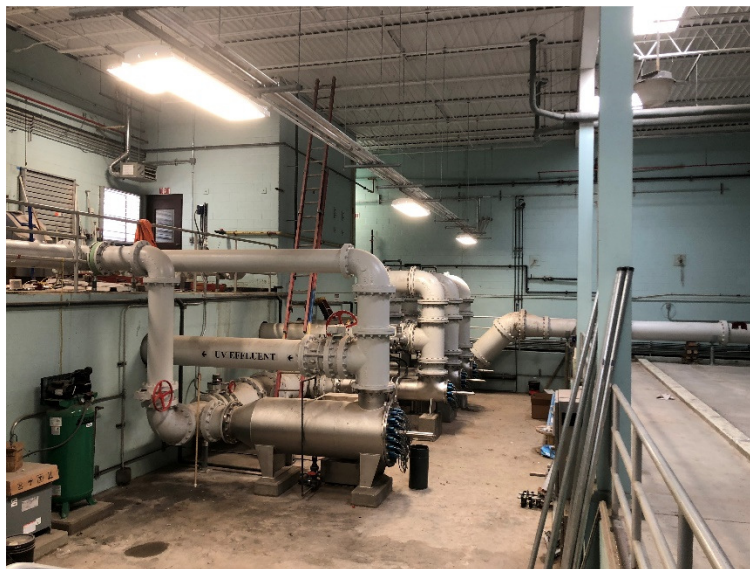
Figure 5-7: Closed Vessel UV Disinfection System
