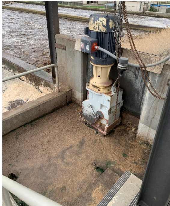
Figure 2-8: Aeration Basin Flooded Gearbox Platform
