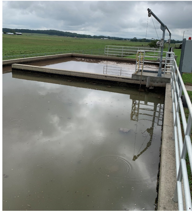
Figure 2-6: Anaerobic Selector Cells 2 & 3
