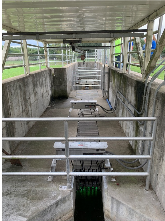
Figure 2-13: Open Channel UV Disinfection System
