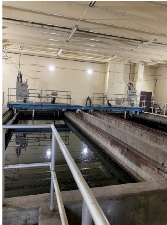
Figure 2-12: Tertiary Sand Filters 1 and 2
