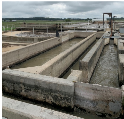
Figure 2-5: Existing Grit Chamber
