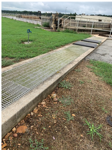
Figure 2-7: Anaerobic Selector Overflow Channel
