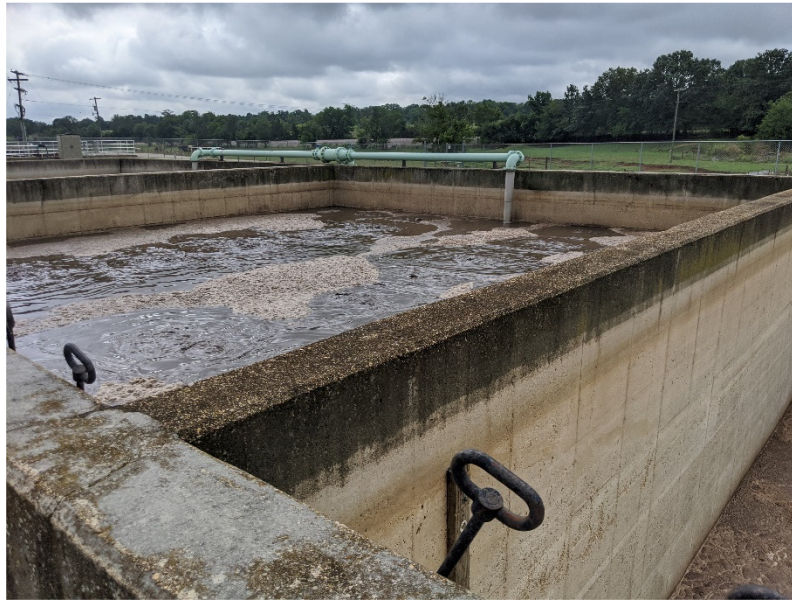
Figure 2-14: Aerobic Digester with Diffused Aeration
